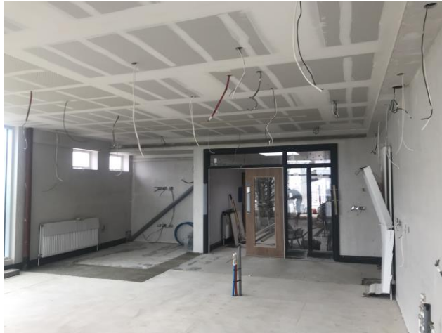
Inside the newly extended Coffee Bar
