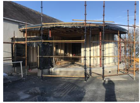
The Entrance Foyer
