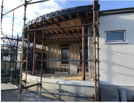
The Entrance Foyer
